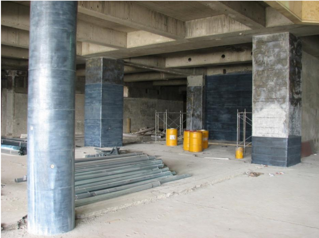
Interior RC columns are strengthened by Carbon Fiber CFRP Composite. 04/15/2008
