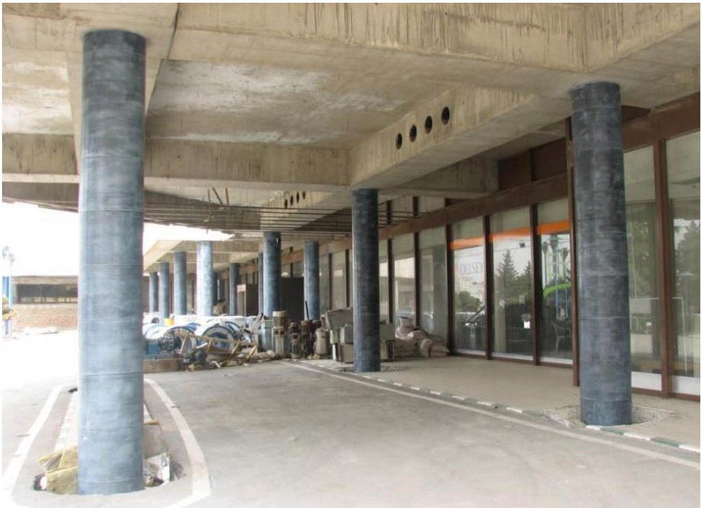
Exterior columns are strengthened by Carbon Fiber CFRP Composite. 04/15/2008
