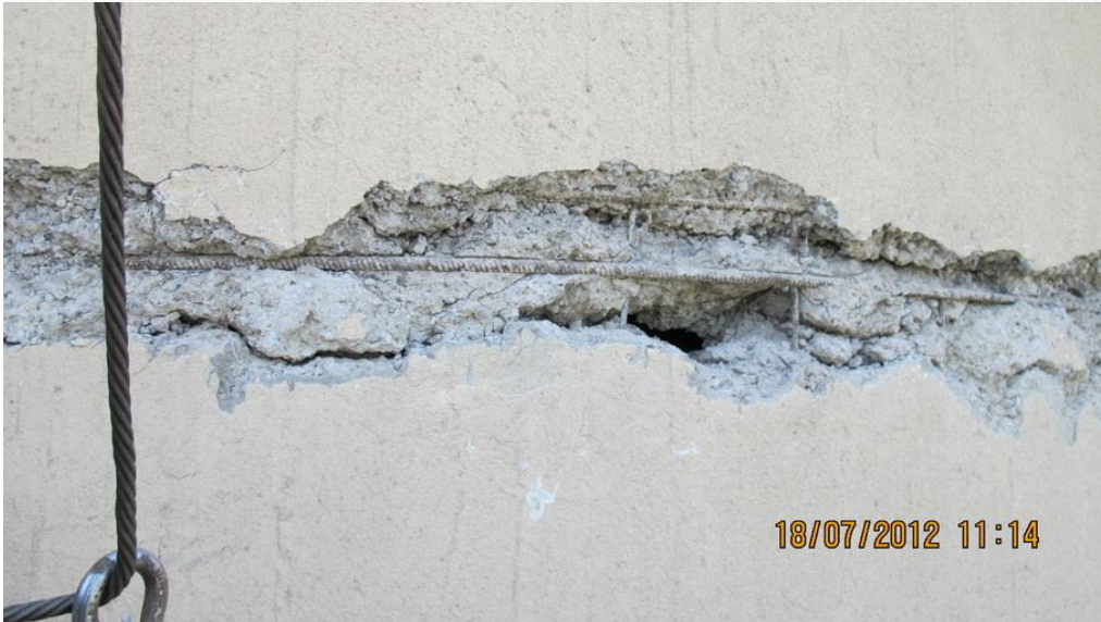
Horizontal crack is so deep to let rain fall penetrate inside the silo.
