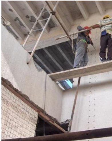
Implanting rebars in the elevator walls to establish new RC concrete shear walls to resist earthquake lateral force. Mohammadi Hospital, Bandar Abbas, Iran 04/18/06
