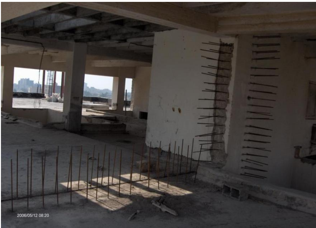
Implanting rebars in the decks and walls to establish new RC concrete shear walls to resist earthquake lateral force. Mohammadi Hospital, Bandar Abbas, Iran 04/20/06
