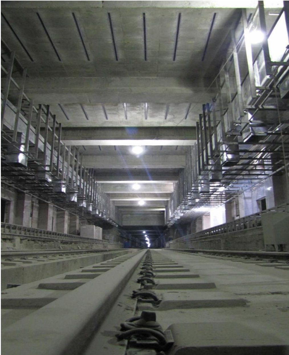
A beautiful view: CFRP Carbon Fiber Stripes are applied under the RC slabs to increase their flexural capacity. Ehsan Station, Shiraz Metro, Shiraz, Iran
