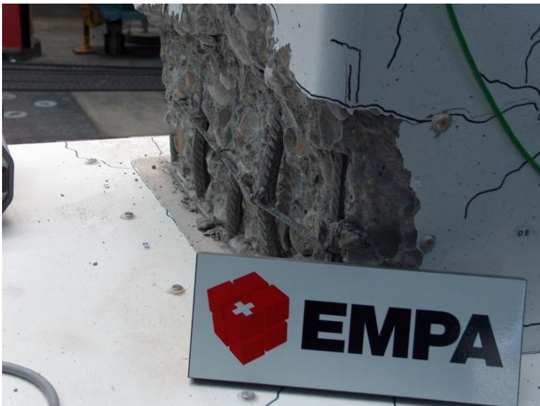
Test results shows compression rebars buckling under bending loads. Empa structural labs, Zurich, Switzerland 07/20/2005
