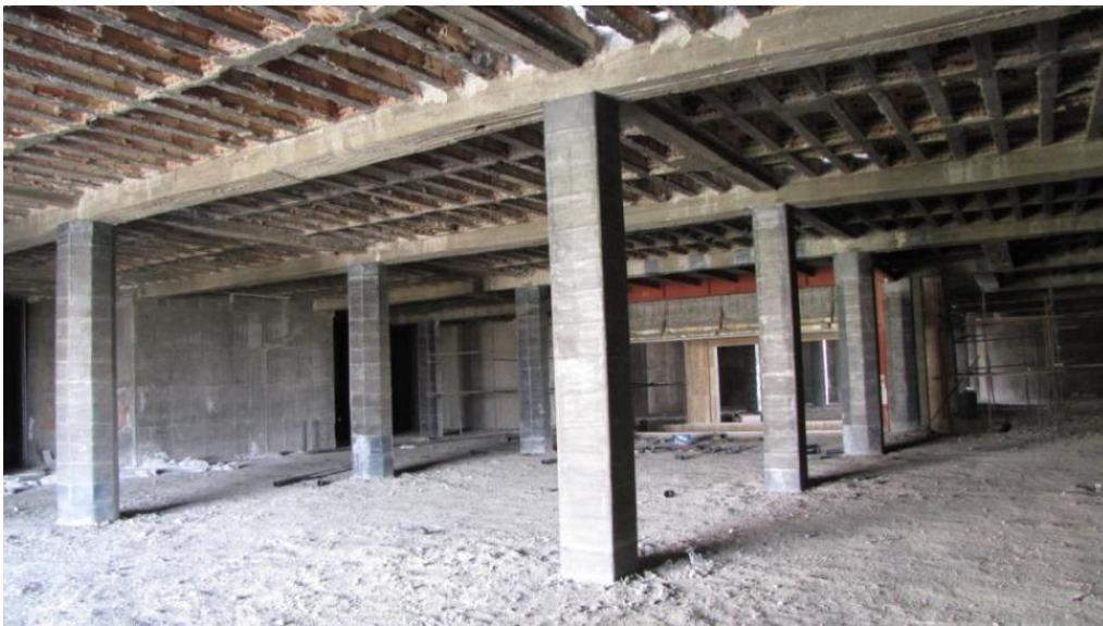
Shear strengthening of the RC beams is completed. Tehran, Iran 07/16/2008
