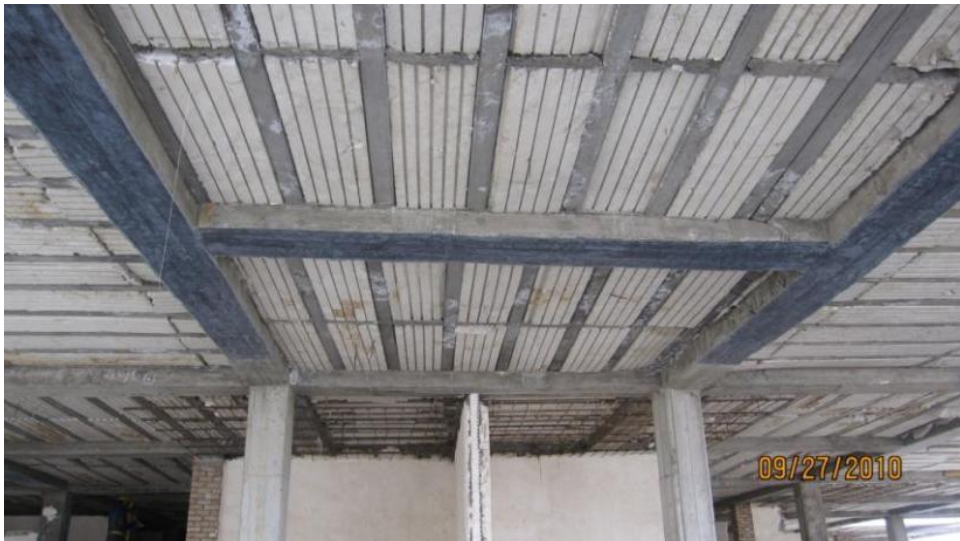
Above Pictures: CFRP Sheets are applied beneath the beams to increase their bending capacity. Radyab Co., Meshkinshahr, Ardebil, Iran
