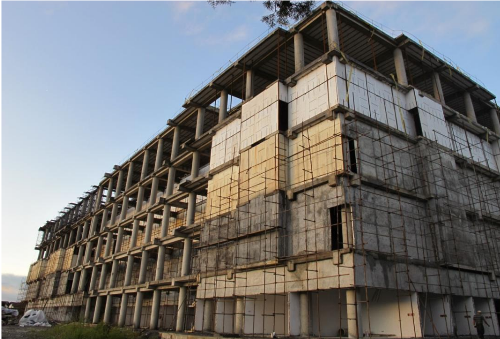
Adine Shopping Centre under construction.
