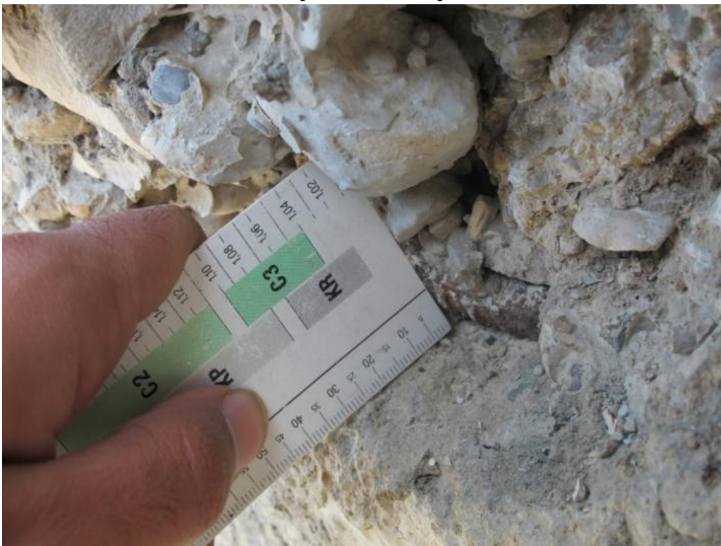
Close view of the crack shows depth of the crack and its porosity.
