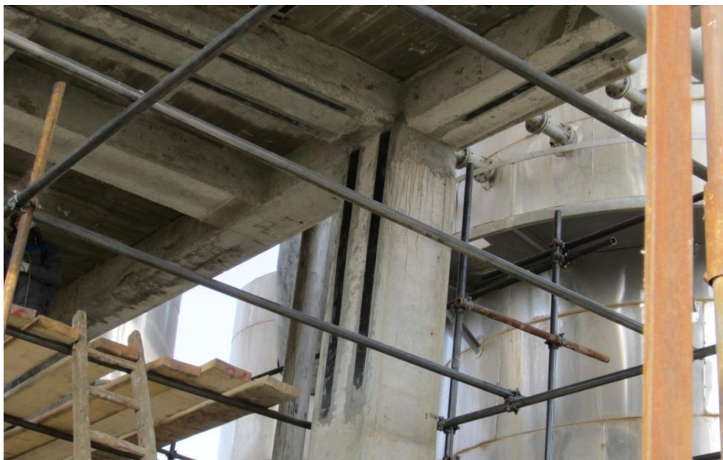
Above Pictures: Installation of carbon fiber stripes on the RC beams and columns in Kimiadaran plant to upgrade load capacity of the structure.
