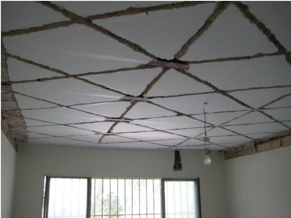
Steel Bracings provided to improve the floor deck's consistency. Tehran, Iran 06/13/2008
