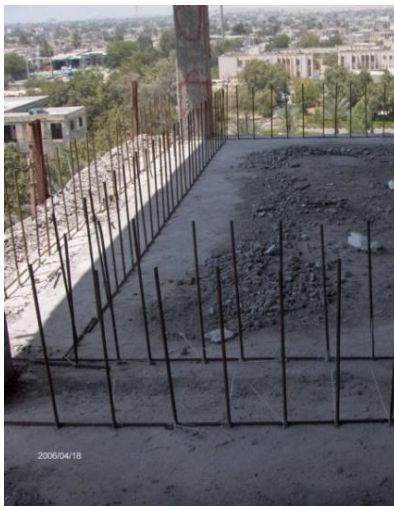
New reinforcement builds up on the implanted rebars to establish new RC concrete shear walls. Mohammadi Hospital, Bandar Abbas, Iran 04/18/2006
