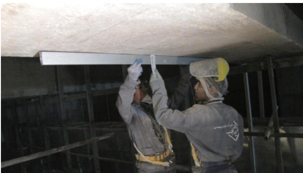
Grinding the concrete beam surface and substrate preparation before applying the CFRP Strips. Ehsan Station, Shiraz Metro, Shiraz, Iran
