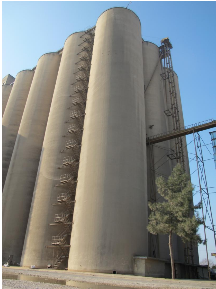
Neka Wheat Silos consisting of 33 concrete silos of 50 meter height, Neka, Iran 2012
