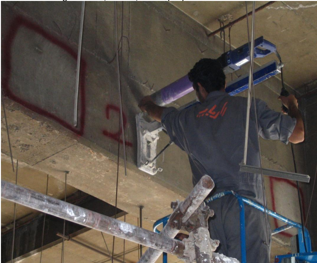
Destructive Tests (concrete core) on the RC beams to evaluate the existing structure material properties. Radyab Co., Esteghlal Hotel, Tehran, Iran 11/02/2005
