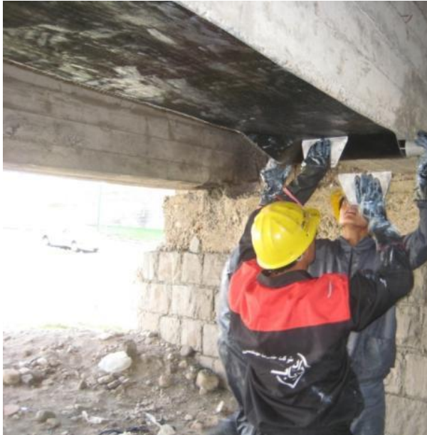
The RC damaged beams are repaired and strengthened by CFRP sheets.
