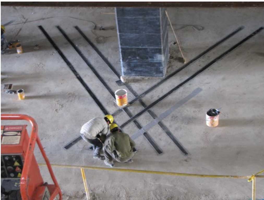
A CFRP wrapped column and diagonal CFRP stripes on the concrete deck for bending strengthening of beams. Khalij Fars shopping Mall, Shiraz, Iran 04/19/2010
