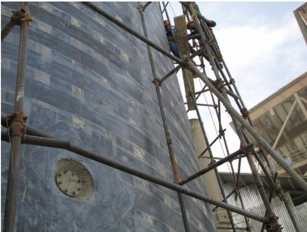
CFRP Sheets used for retrofitting the Abaadeh cement factory silos, Abaadeh, Fars Province, Iran 2010 - 2011
