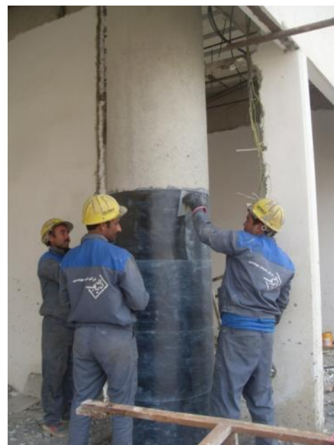
Radyab Co. personnel are grinding and then wrapping the columns with FRP composites.
