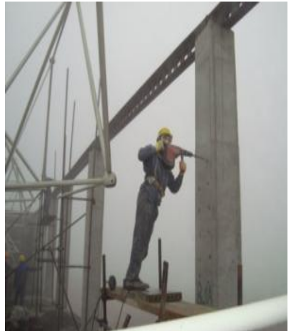
Surrounding columns are drilled based on the structural strengthening design for implanting steel bars in Concrete Jacketing method.
