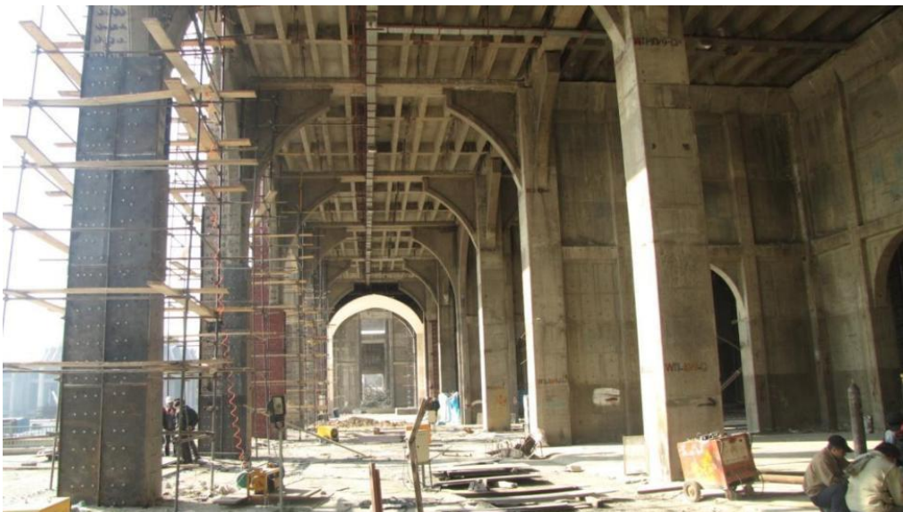
Above Pictures: Exterior and Interior view of the RC columns to be strengthened.
