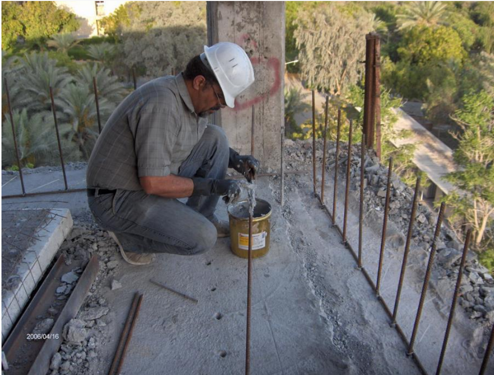
Implanting rebars in the floor decks to establish new RC concrete shear walls to resist earthquake lateral force. Mohammadi Hospital, Bandar Abbas, Iran 04/16/06
