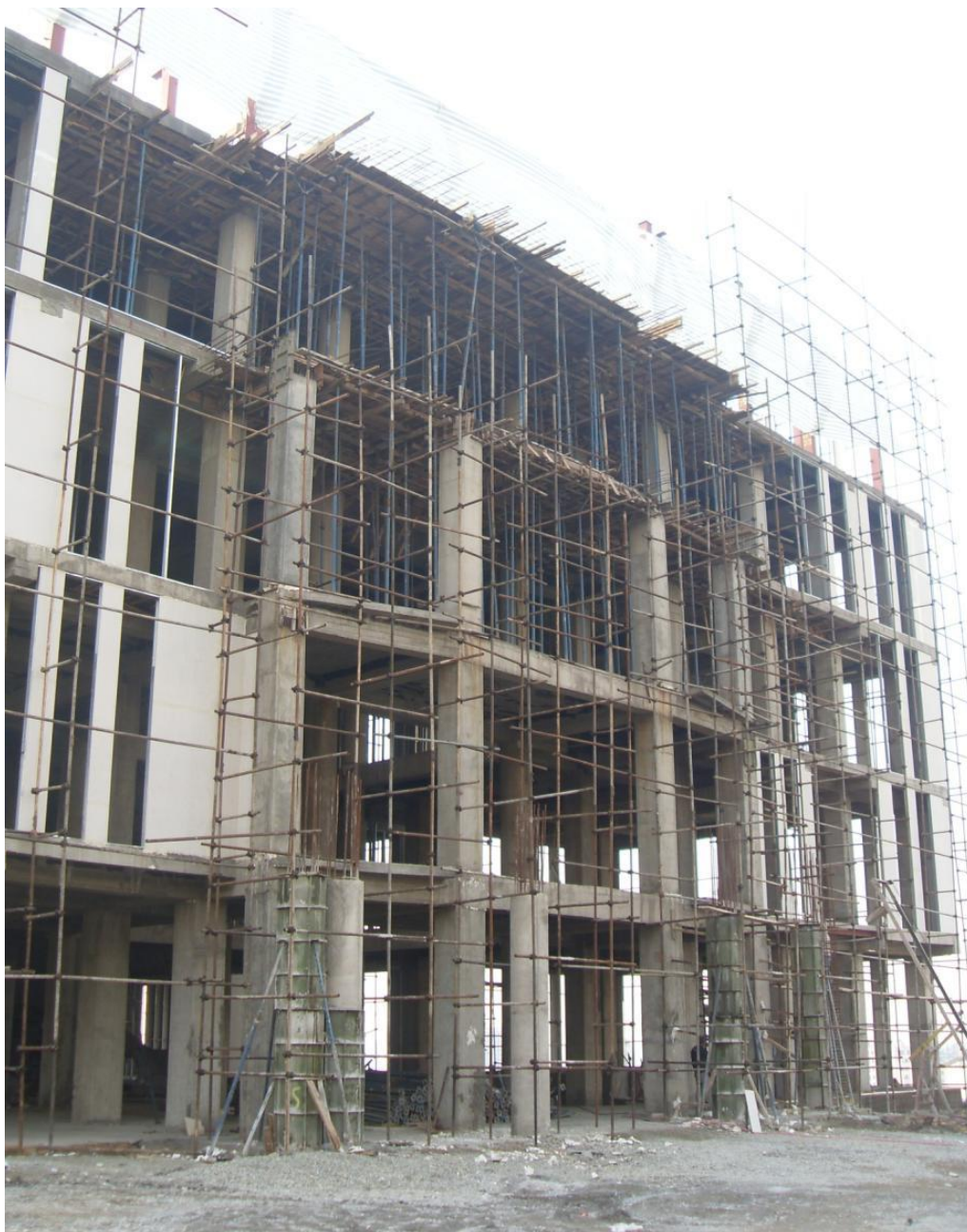
Seoul official building under construction, Tehran, Iran.
