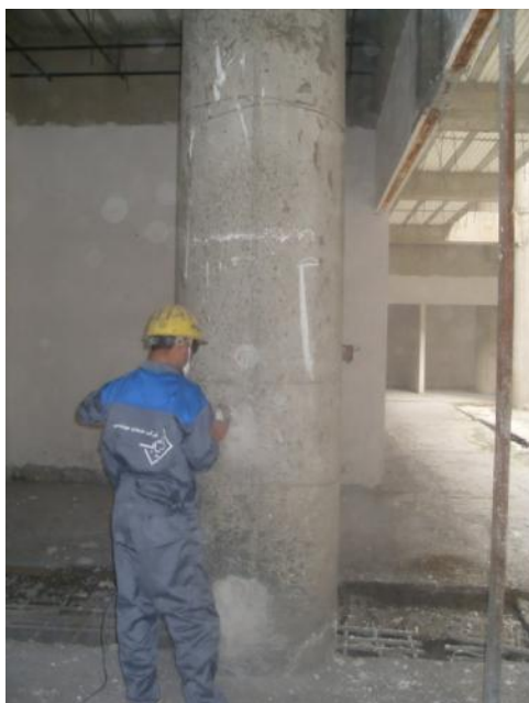
Radyab Co. personnel are grinding and then wrapping the columns with FRP composites.
