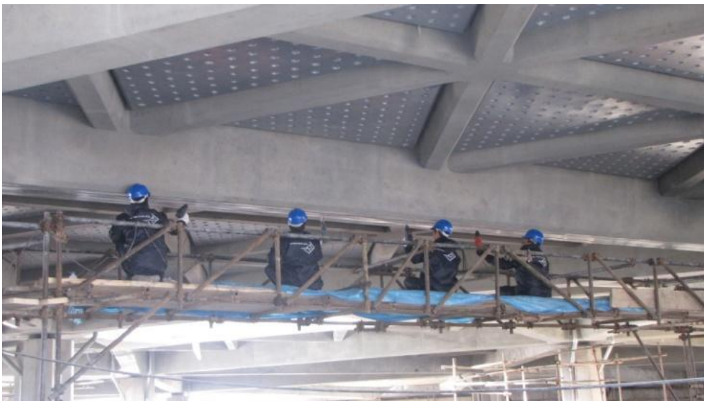
CFRP Carbon Fiber stripes are being applied under the RC beams using a high platform to allow the traffic pass underneath. Qom, Iran 01/28/2010
