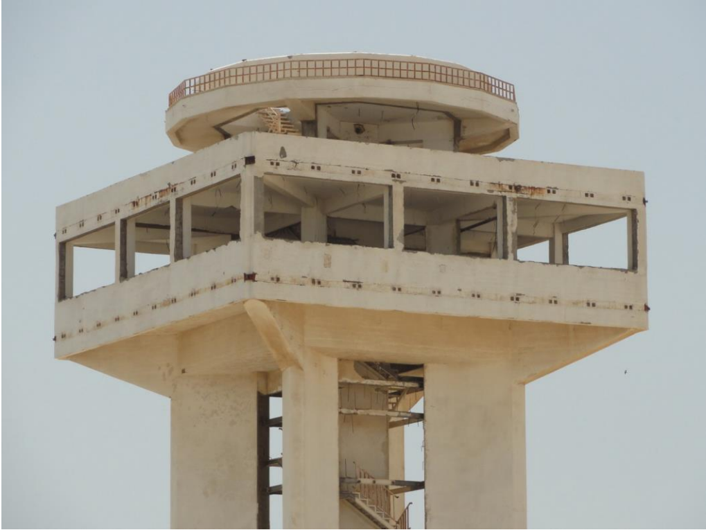
The control room was separated from the main structure due to earthquake
