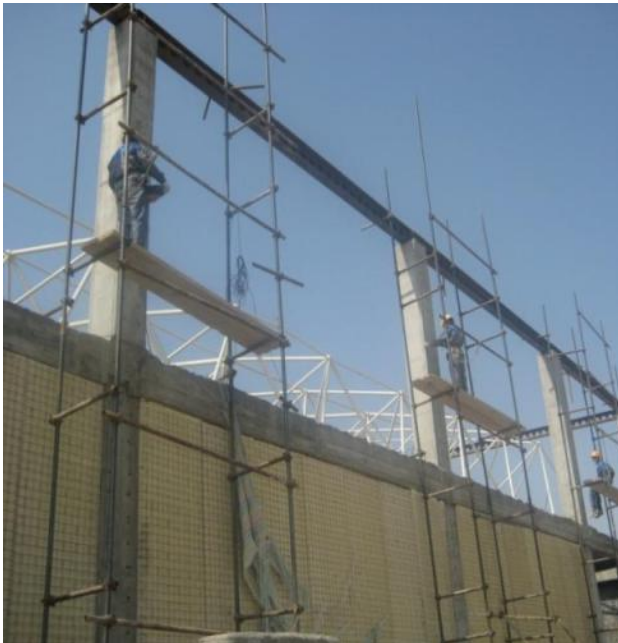
Surrounding columns are drilled based on the structural strengthening design for implanting steel bars in Concrete Jacketing method.
