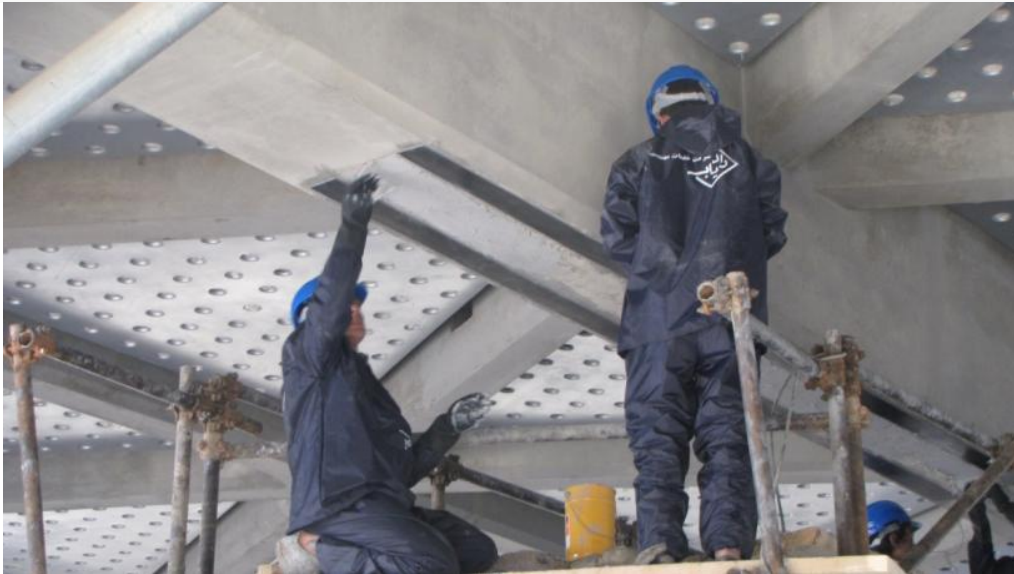
Radyab Staff is applying CFRP Carbon Fiber stripes under the RC. Qom, Iran
