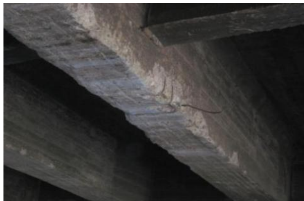
Above and front pictures: The RC bridge and some of the damaged beams before being repaired and retrofitted
