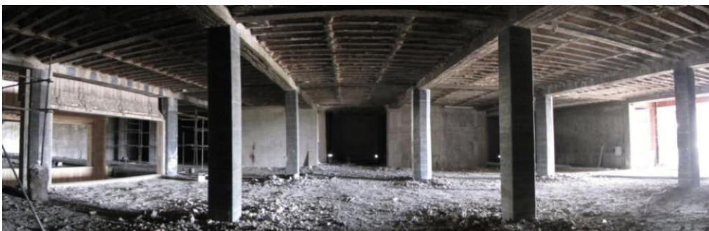
All of the old RC columns are strengthened by CFRP Carbon Fiber column wrapping method in the above pictures. Tehran, Iran 11/06/2007
