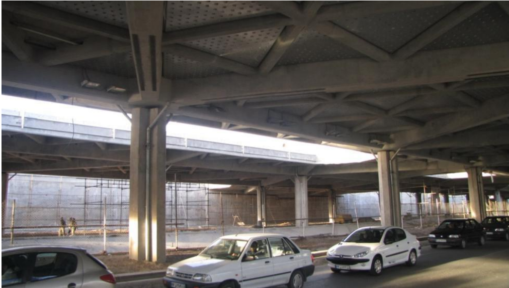
CFRP Carbon Fiber stripes are installed under the RC beams to meet the local rebar overlap demand. Qom, Iran 10/18/2009
