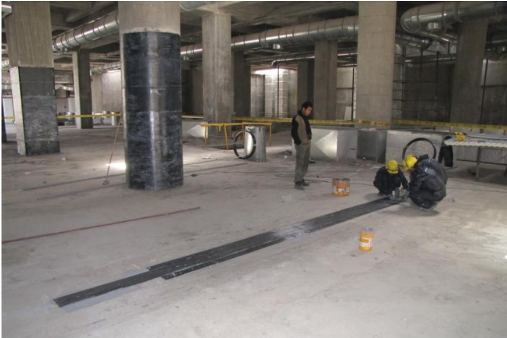
Columns and beams are being strengthened by Carbon Fiber CFRP Composites by Radyab Co., Khalij Fars shopping Mall, Shiraz, Iran 03/11/2010
