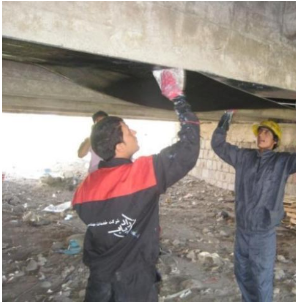
The RC damaged beams are repaired and strengthened by CFRP sheets.
