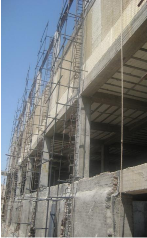
Surrounding columns bending capacity is increased by Concrete Jacketing method. Golestan shopping center. Radyab Co., Meshkinshahr, Ardebil, Iran
