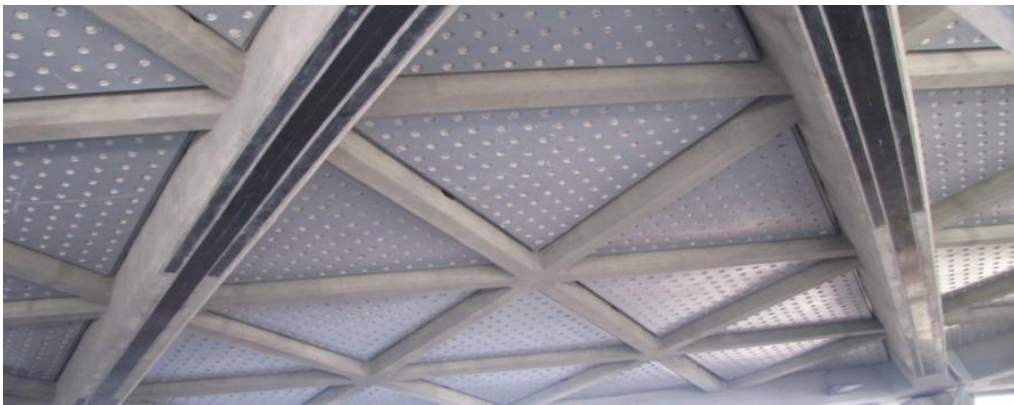
Two lateral CFRP Carbon Fiber stripes are applied under the RC beams to meet the local rebar overlap demand and the two additional stripes in the middle are to provide total consistency of the beam. Qom, Iran 01/28/2010
