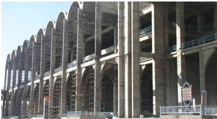
Above Pictures: Steel Jacketing starts with drilling holes to implant steel bolts inside them by means of special high strength Epoxy Resins.
