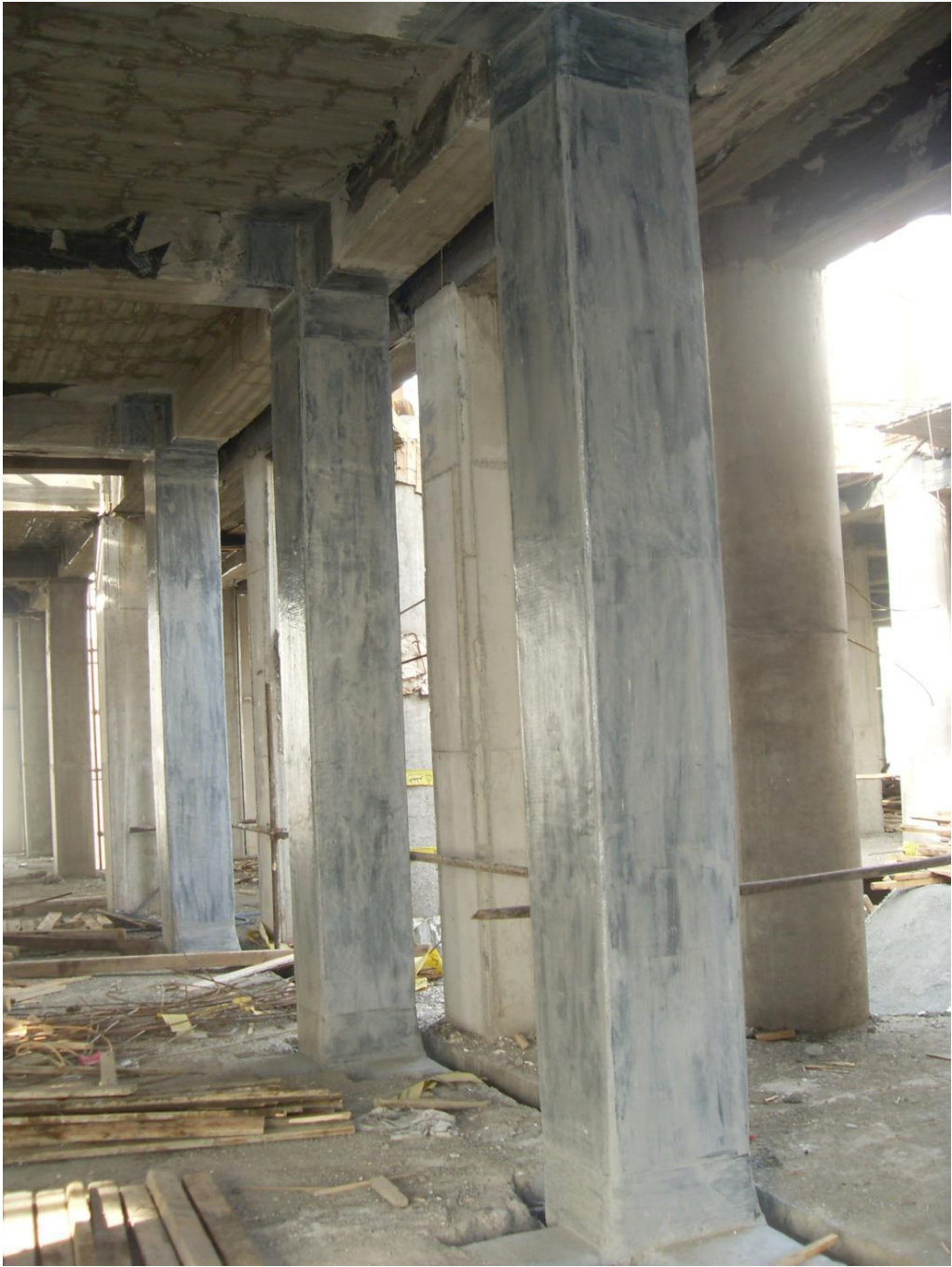
Columns are strengthened for bending at their overall length.
