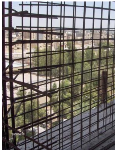
New reinforcement builds up on the implanted rebars to establish new RC concrete shear walls. Mohammadi Hospital, Bandar Abbas, Iran 04/18/2006
