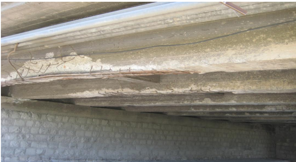
Above and front pictures: The RC bridge and some of the damaged beams before being repaired and retrofitted
