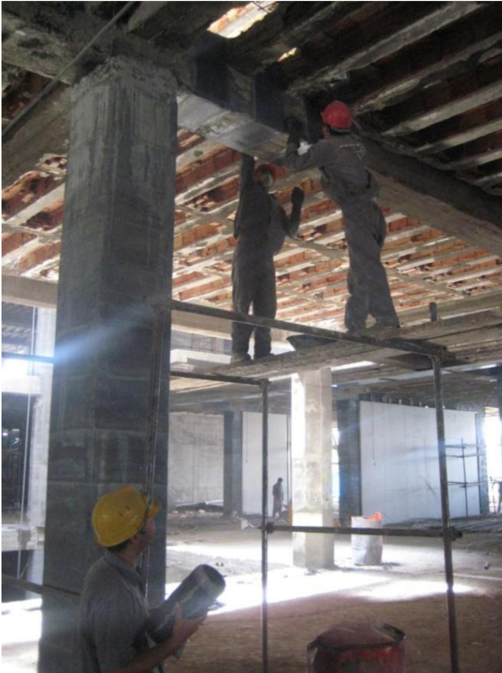
CFRP Carbon Fiber Sheets are applied on the RC beams to upgrade their Shear Stress capacity. Tehran, Iran 07/16/2008
