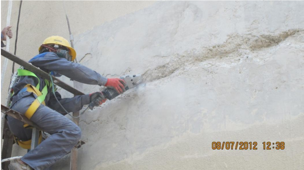
Above Pictures: Radyab Co. personnel are repairing the concrete substrate by means of grinding before the application of CFRP fabrics.
