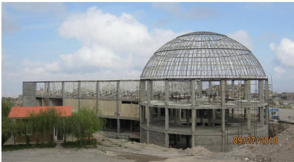
Installation of space frame in Golestan Shopping Centre, Meshkinshahr, Ardebil, Iran.
