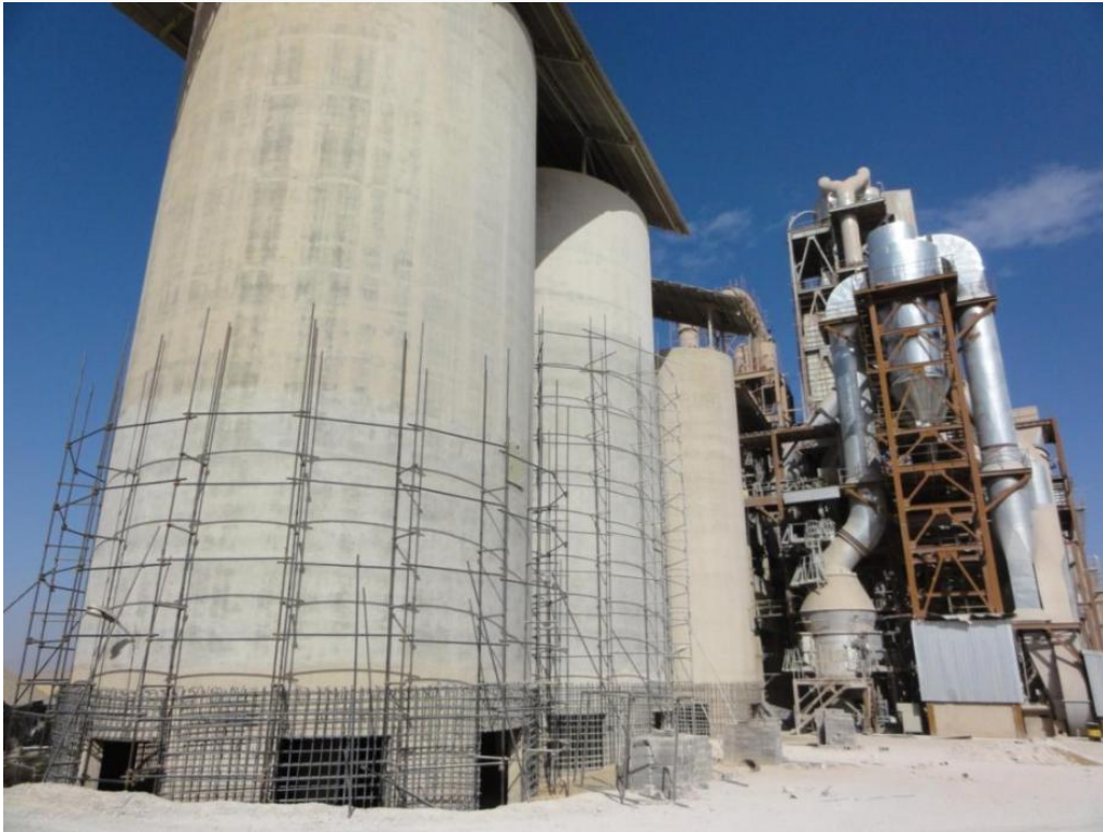
Grinding the concrete surface as the first step of structural strengthening before repairing the concrete.
