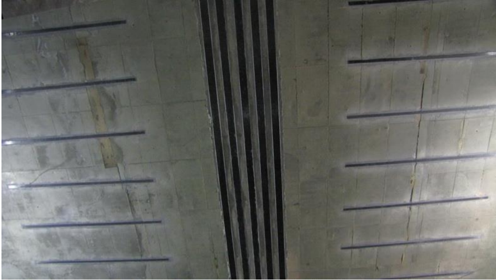
The main beams are strengthened by means of 5 high modulus Carbon Fiber Laminates of 10 Cm width and 1.4 mm thickness. Ehsan Station, Shiraz Metro, Shiraz, Iran
