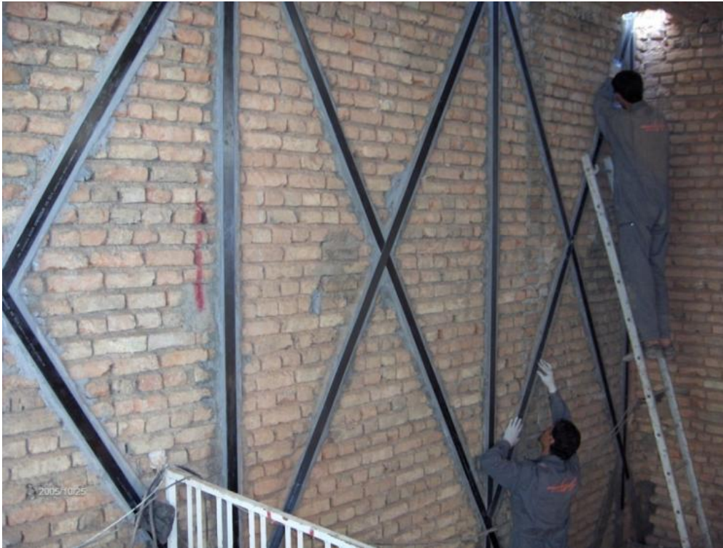
Radyab Co. staff applying CFRP stripes on the masonry walls. Shariati Museum, Tehran, Iran, 10/05/2005
