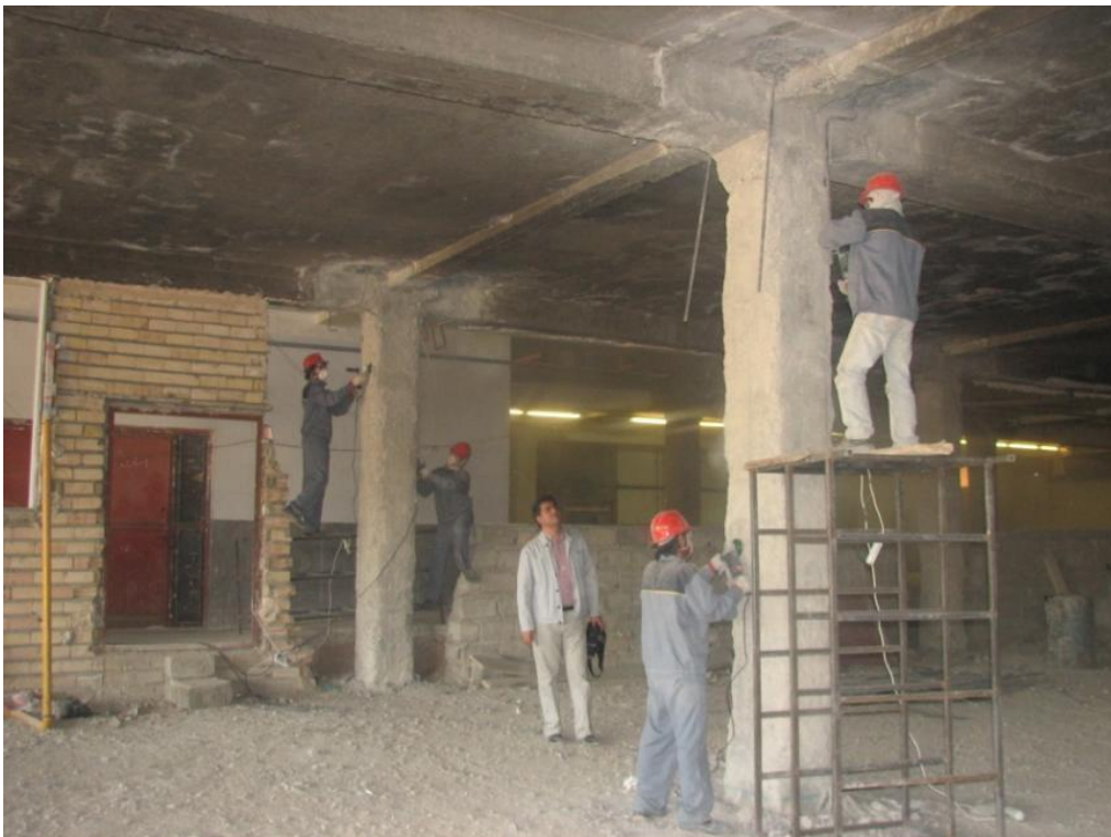
Radyab staff grinding the surface of the RC columns to prepare them for retrofitting by wrapping CFRP fabrics. Mr. Javad Najafi (middle) is supervising. Tehran, Iran 11/06/2007
