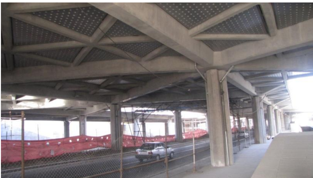
Traffic is running under the bridge during strengthening work. Qom, Iran 02/21/2010
