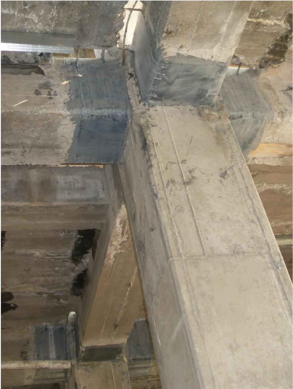
Beams are strengthened for shear at the ends (supports).
