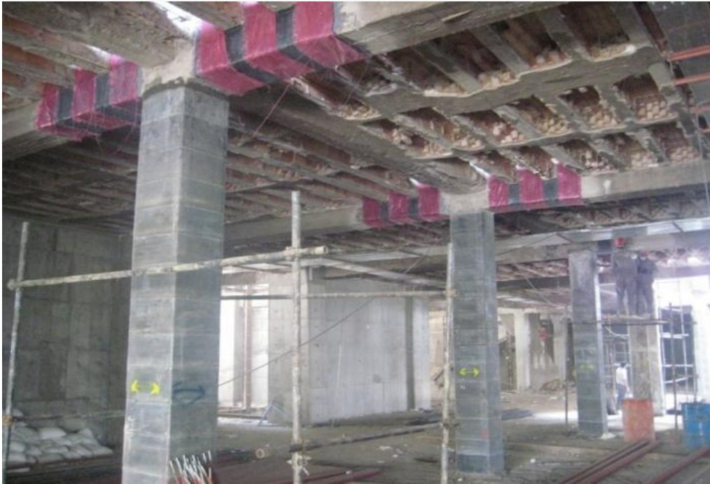
Shear strengthening of the RC beams is completed. Tehran, Iran 07/16/2008
