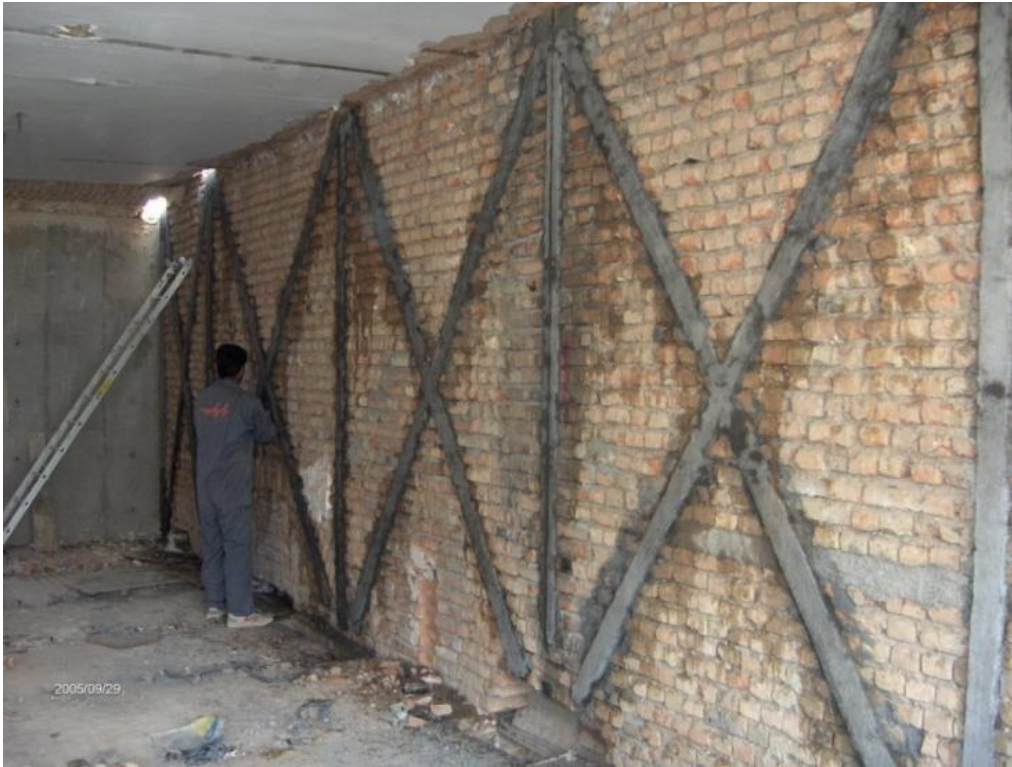
Radyab staff applying high strength repair mortar as substrate for CFRP stripes on the masonry walls. Shariati Museum, Tehran, Iran, 10/05/2005
