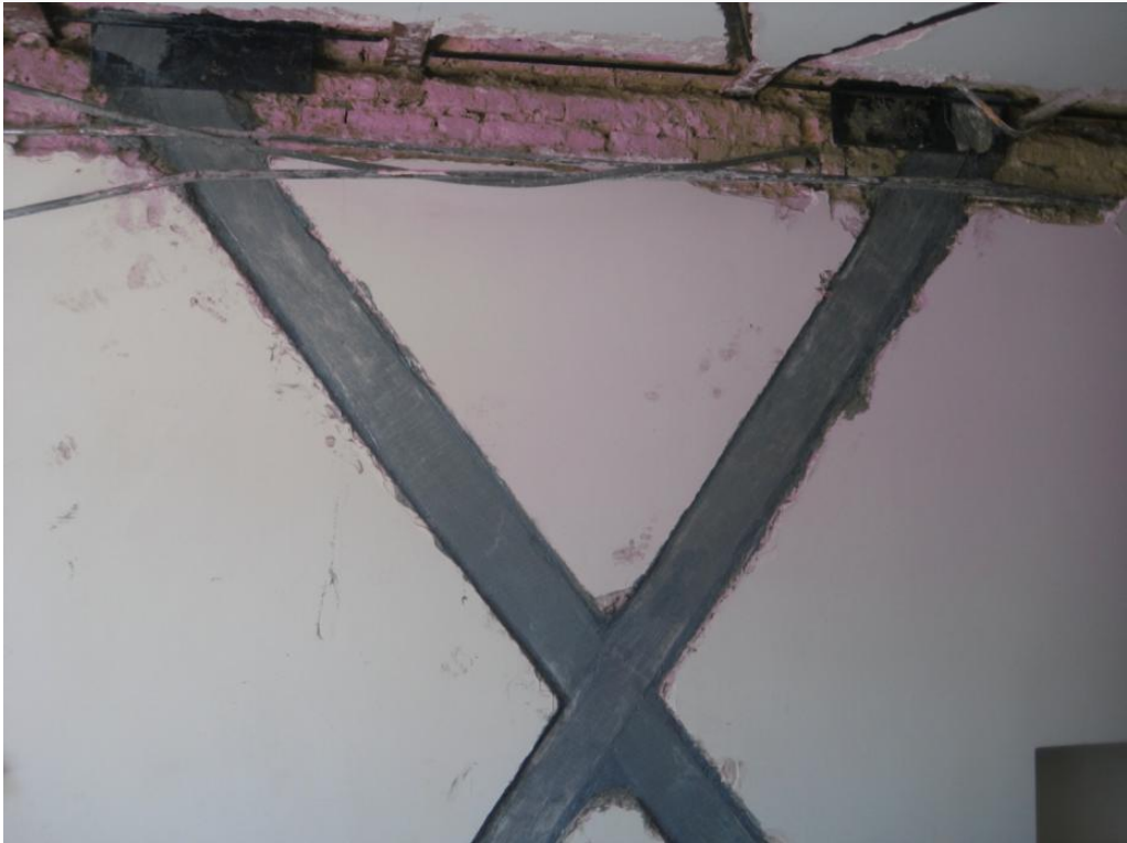
GFRP Composite Bracings to protect the masonry walls from out of plane bending. Tehran 10/19/2008
