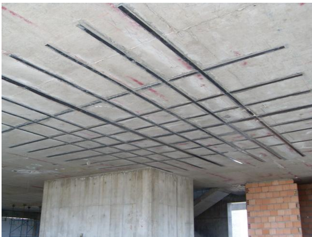
Carbon fiber strips are installed at the bottom side of the deck in X and Y axes.
