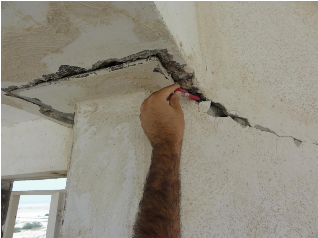
Above Pictures: Damages to the Qeshm International Airport Control Tower due to 2012 earthquake
