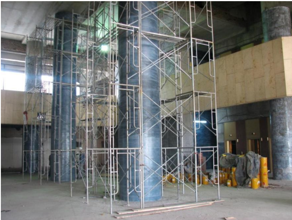
Azadi Grand Hotel Lobby. Main RC columns at the middle of the lobby are wrapped by Carbon fiber CFRP composites. Tehran 04/15/2008
