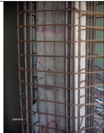
New reinforcement builds up on the implanted rebars to establish new RC concrete shear walls. Mohammadi Hospital, Bandar Abbas, Iran 04/18/2006
