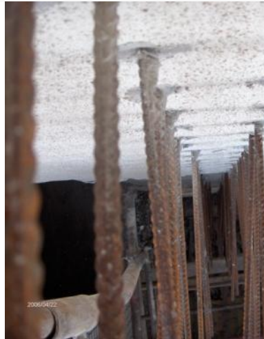
Implanting rebars in the elevator walls to establish new RC concrete shear walls to resist earthquake lateral force. Mohammadi Hospital, Bandar Abbas, Iran 04/18/06
