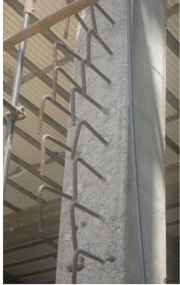
Surrounding columns bending capacity is increased by Concrete Jacketing method. Golestan shopping center. Radyab Co., Meshkinshahr, Ardebil, Iran
