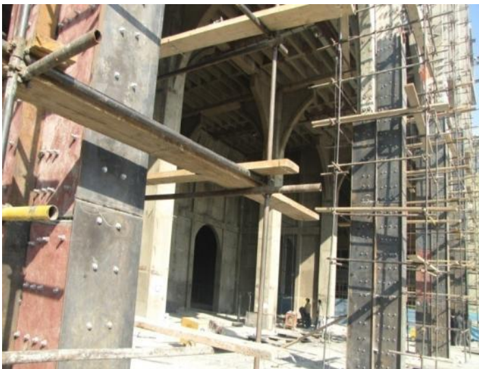
Above Pictures: Implanting steel bolts by means of special high strength Epoxy Resins and then installing the steel sheets are the next steps in this method. Grout injection is the last step to be done after completion of steel sheets welded.
