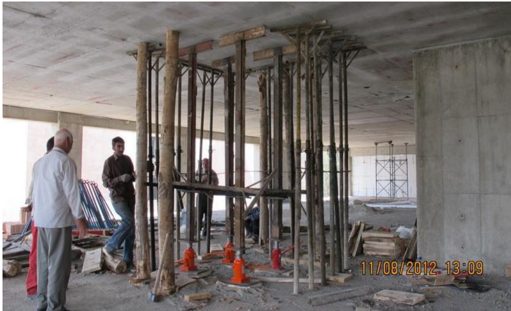
Floor deck is lifted up to compensate the deflection by means of hydraulic jacks.
