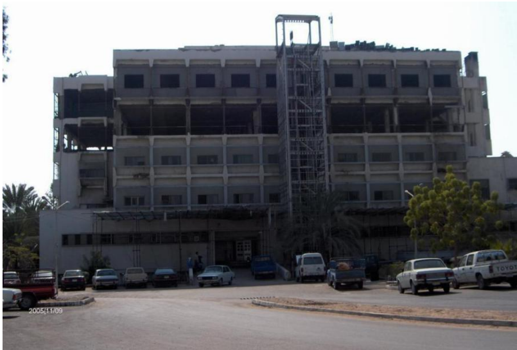
The two upper stories are to be refurbished and renovated while the other floors are operational. Bandar Abbas, Iran 11/09/2005
